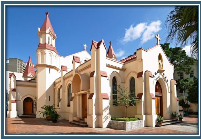
Photo: Rosary Church after renovation in 2003
